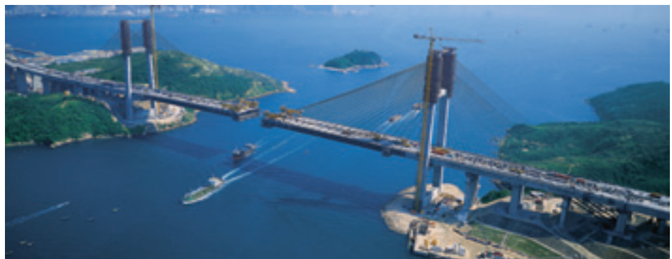
Kap Shui Mun Bridge, Hong Kong
