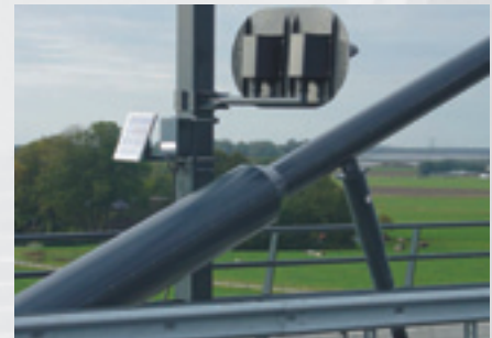
Installed External Damper
